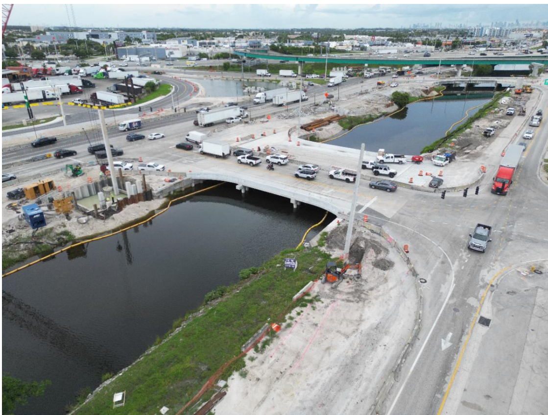
MECHANICALLY STABILIZED EARTH (MSE) WALL ALONG SOUTHBOUND S.R. 826/PALMETTO EXPY. ON-RAMP
