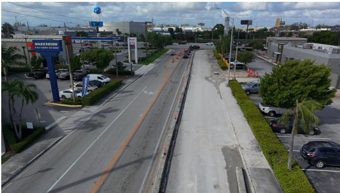
NW 79 AVE BRIDGE
