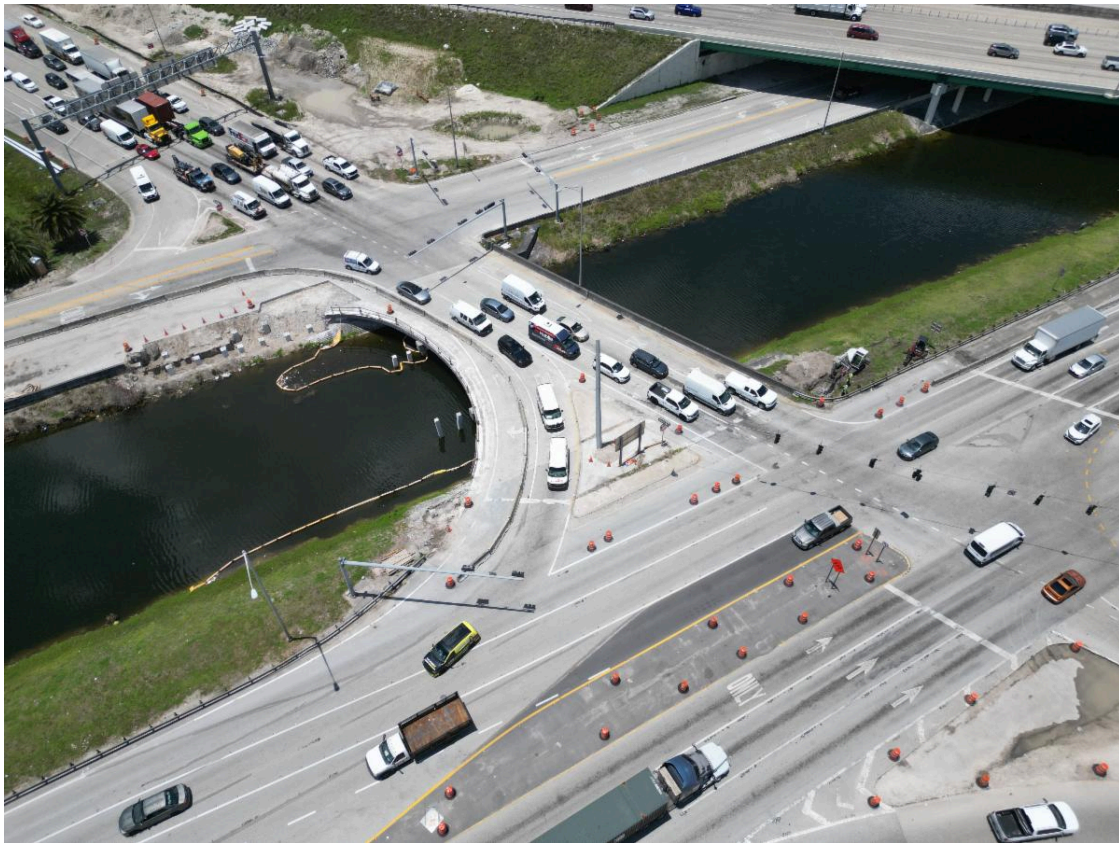
Mechanically Stabilized Earth (MSE) Walls for Ramp B at SB S.R 826/Palmetto Expressway on-ramp
