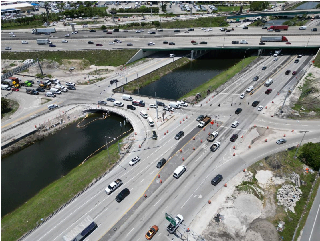
NB S.R. 826/Palmetto Expressway off-ramp Bridge to S.R. 25/U.S. 27/Okeechobee Road
