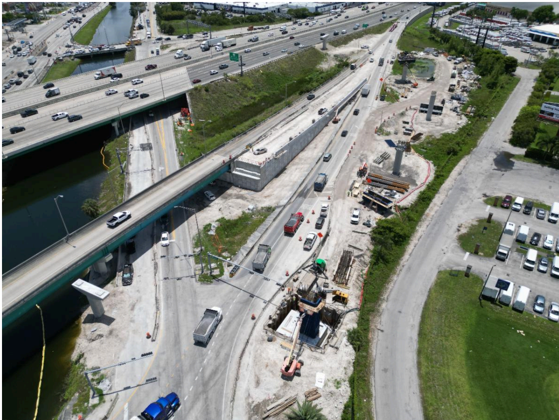
Mechanically Stabilized Earth (MSE) Walls for Ramp B at SB S.R 826/Palmetto Expressway on-ramp
