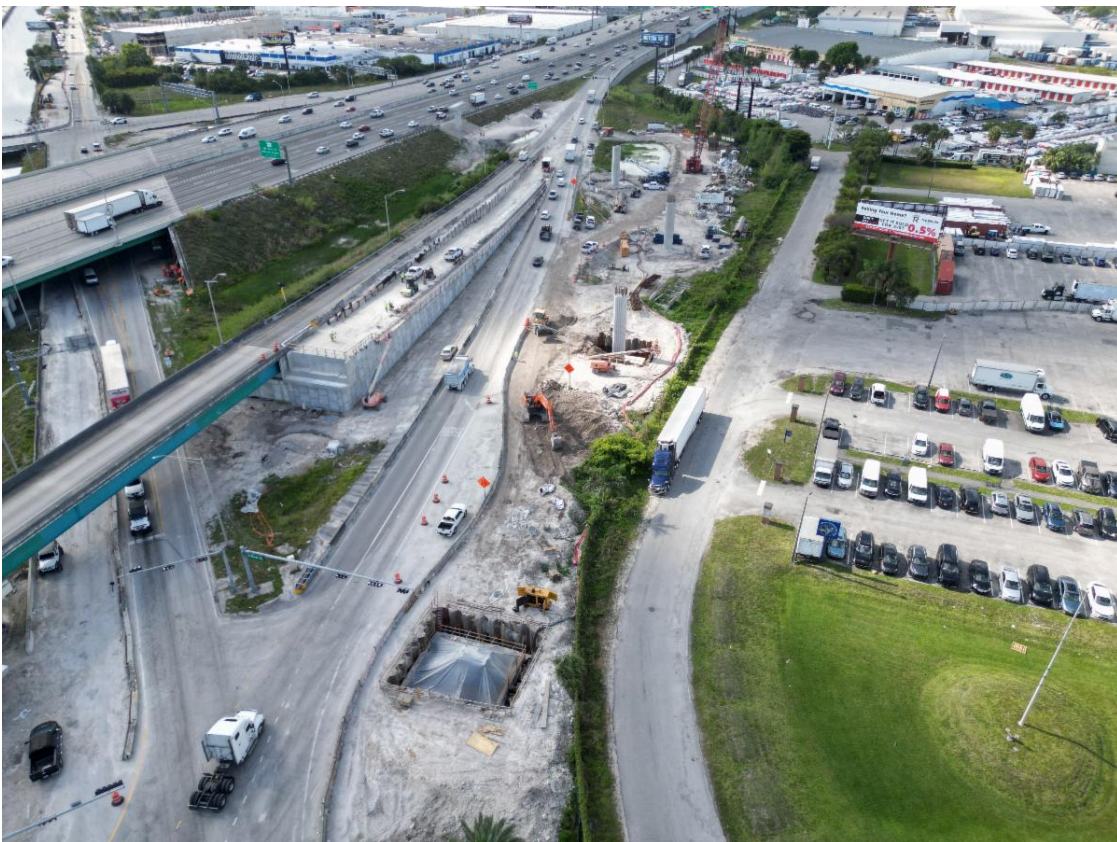
MSE Wall for southbound S.R. 826/Palmetto Expy. on ramp
