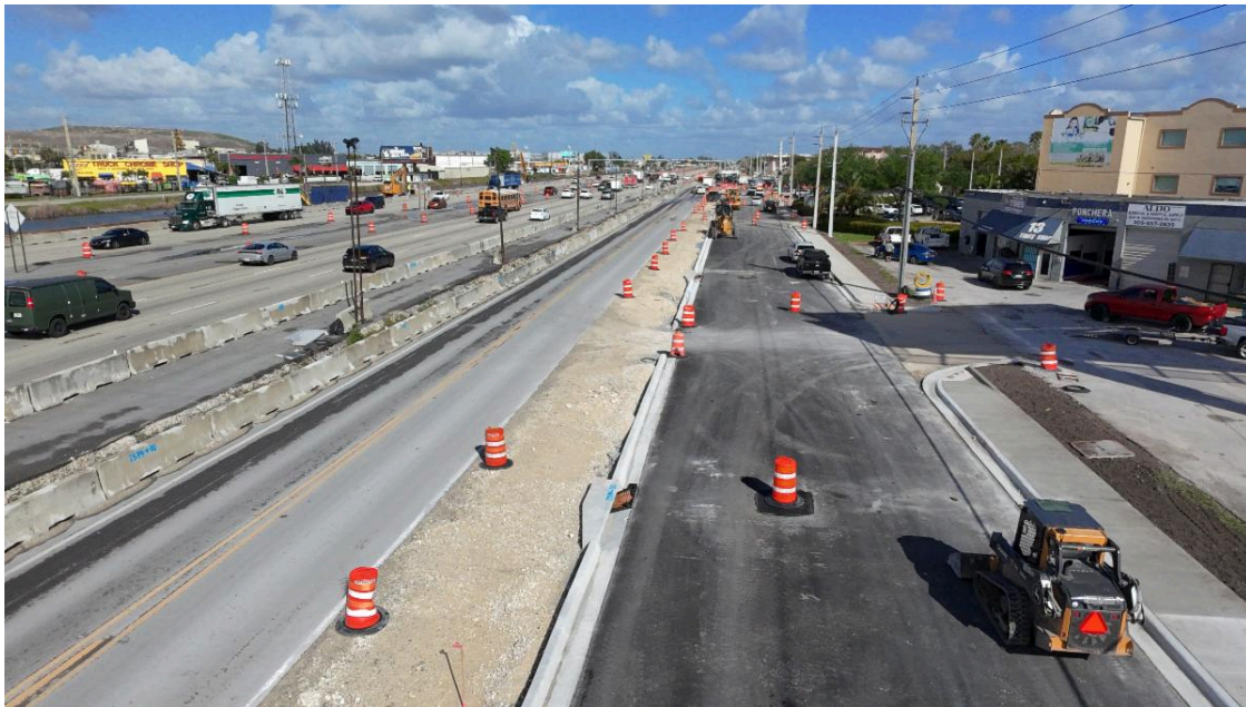
Frontage Road between NW 95 Street and NW 77 Avenue
