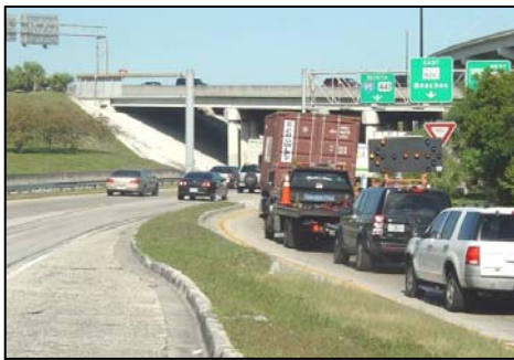
Weaving condition between NB Florida's Turnpike and NB SR 7/I-95
