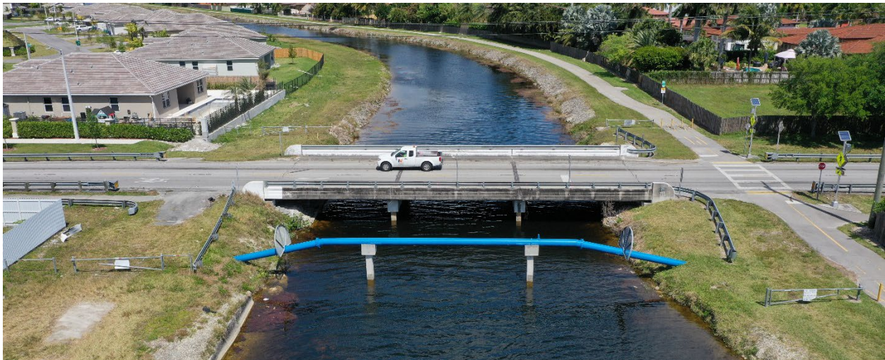
Figure 2-12 Existing Bridge Elevation Looking North
