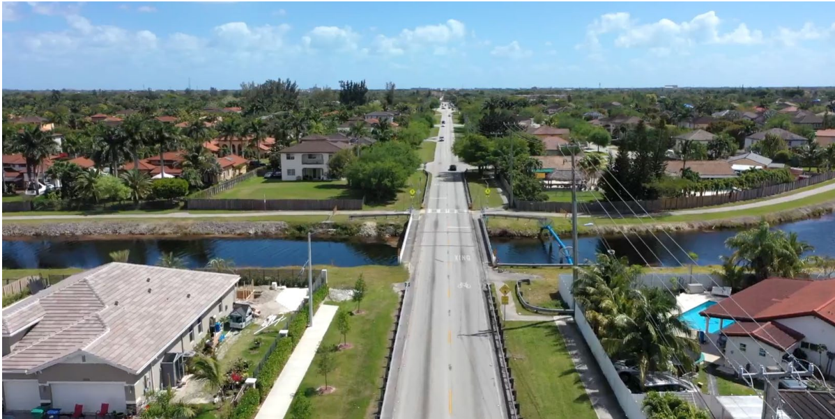
Figure 2-1 SR 994/Quail Roost Drive, west of Black Creek Canal - Looking East
