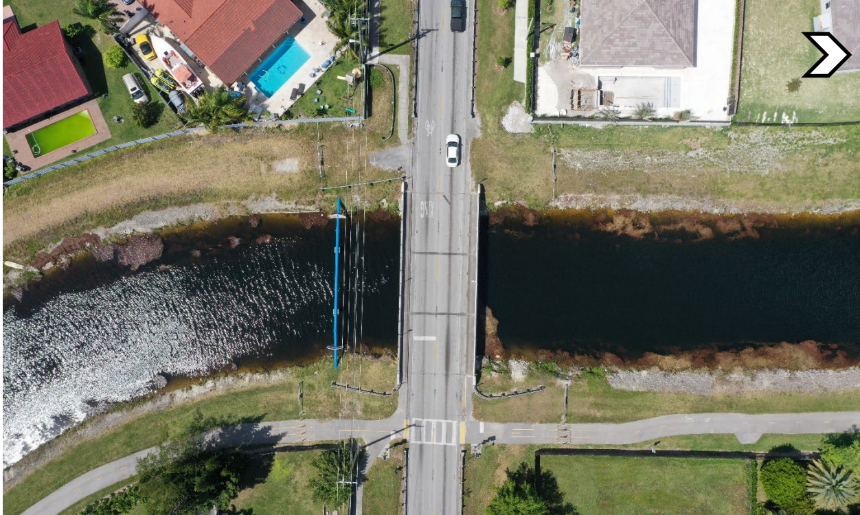
Figure 2-13 Existing Bridge Aerial
