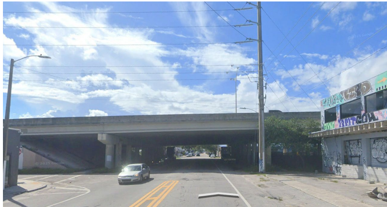
I-95 over NW 71st St.
