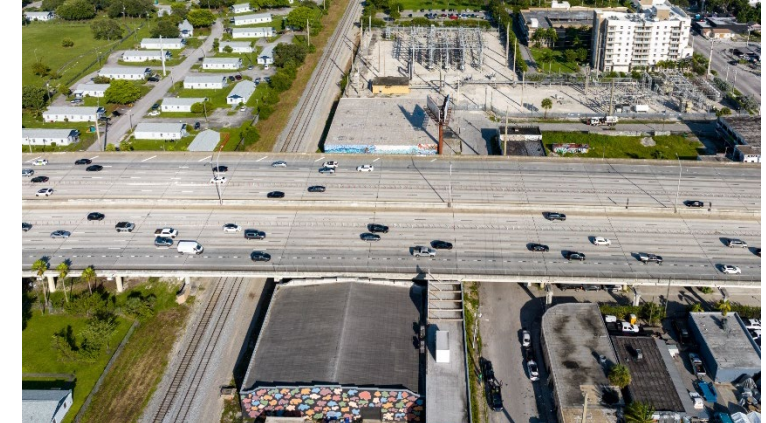
I-95 over Railroad Tracks
