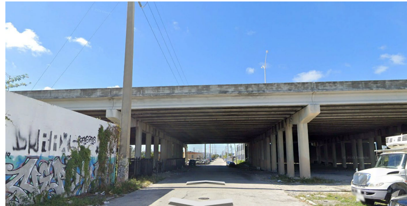
I-95 over NW 72nd St.
