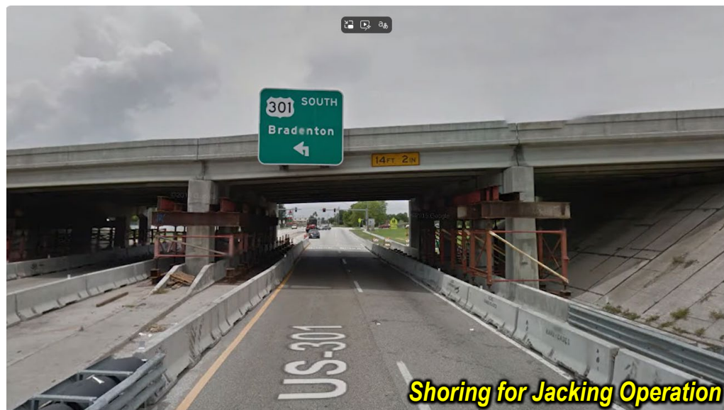
Existing Bridge Raised during Jacking
