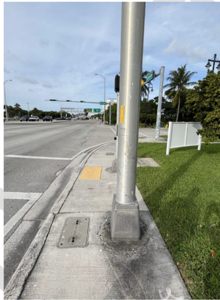
Figure 2.7 | Existing Lighting (SW Corner of NE 79 th Street and Pelican Harbor Drive)
