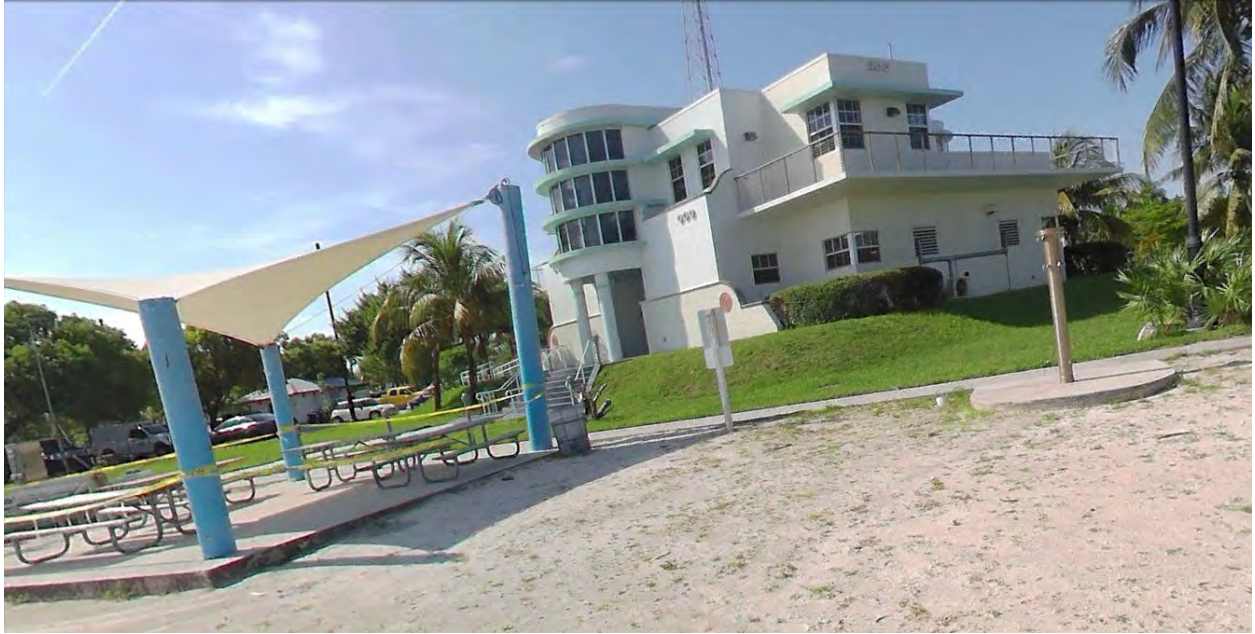
Photo 19 Marina Building and Picnic Area, facing north
