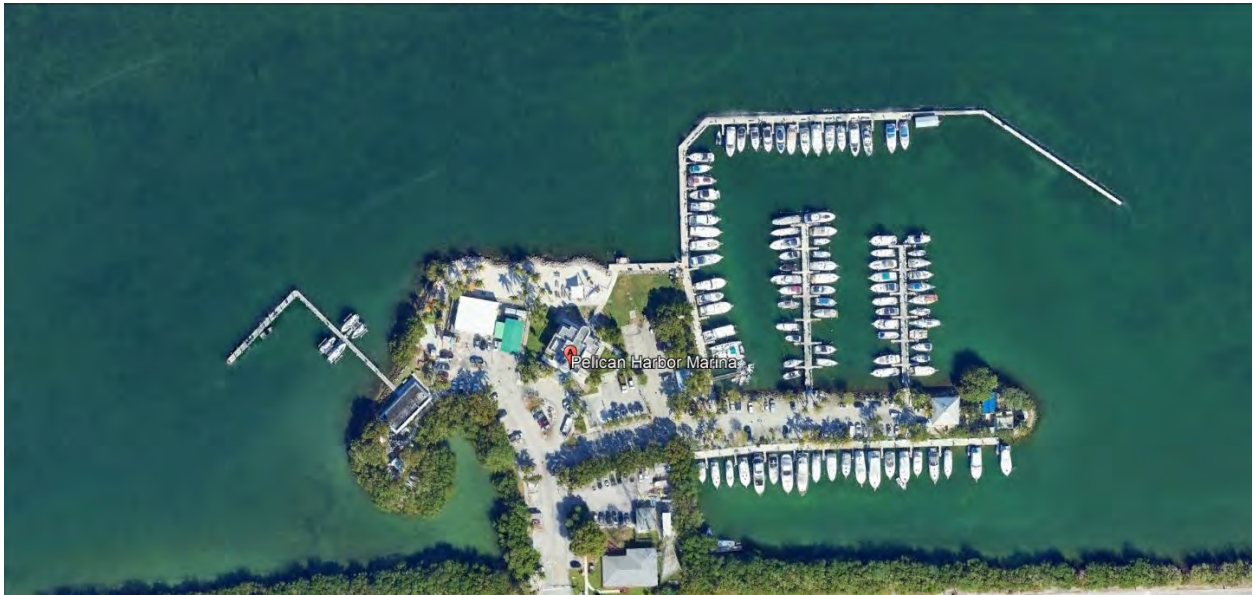
Photo 15 Aerial View of Pelican Harbor Marina
