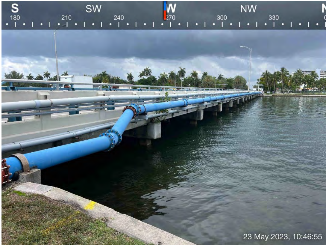
Photo 2 Existing eastern bridge, view from northern limits
