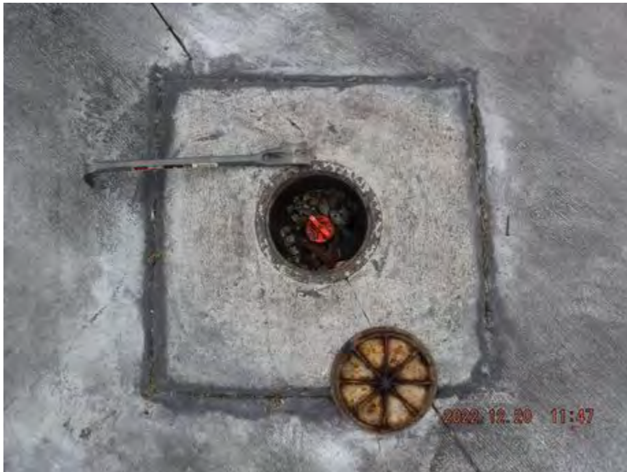
photo 4/4 - top view MW-9 (existing/viable well)
