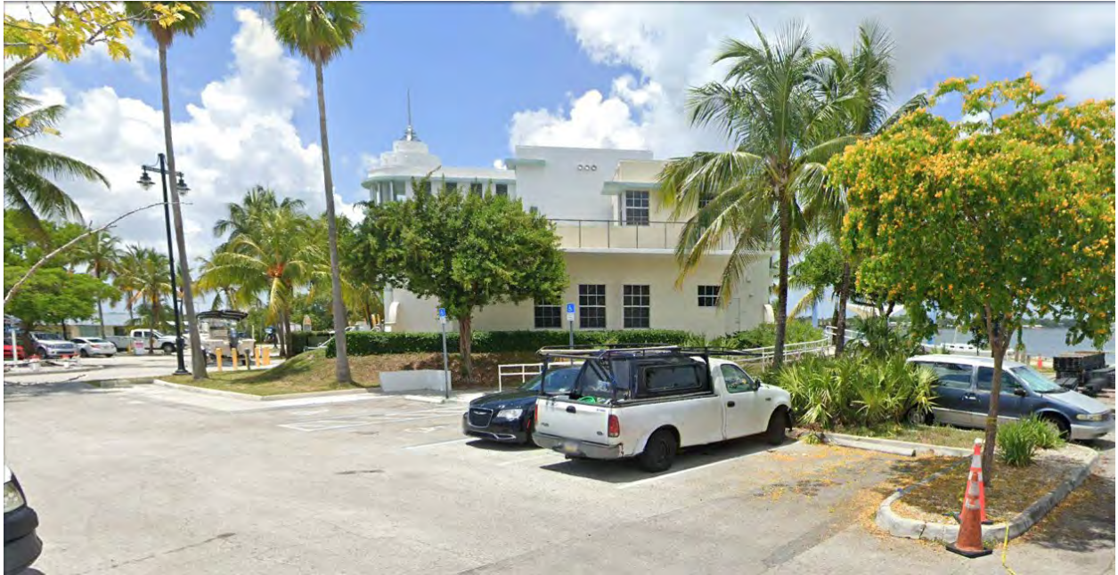
Photo 17 Marina Building, Facing North
