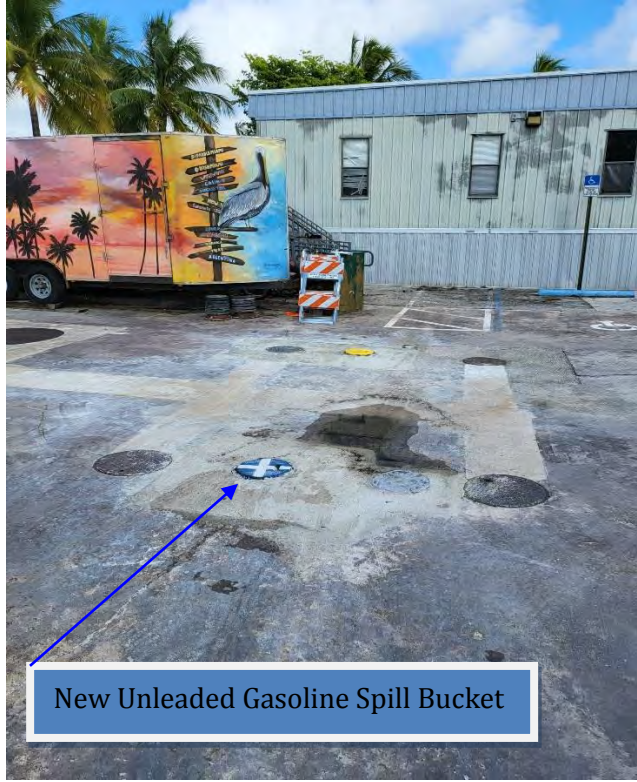
New spill buckets, facing north.
