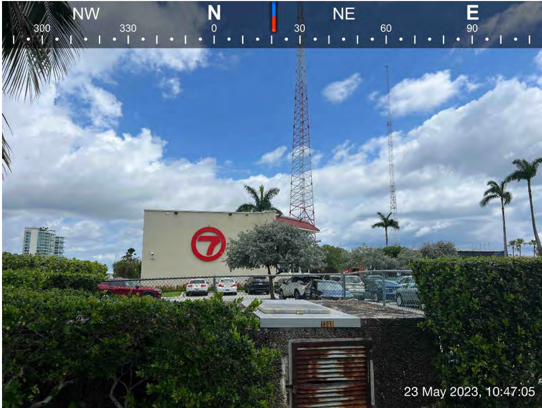
Photo 6 Front of facility
