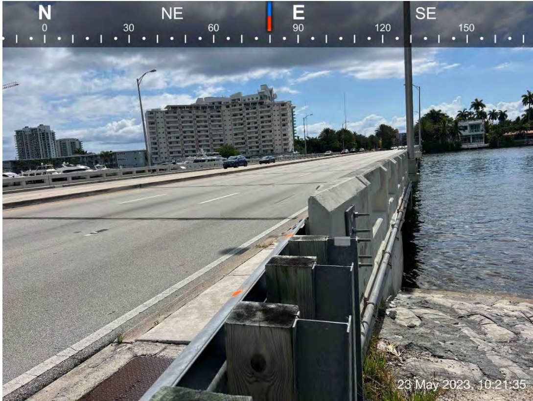
Photo 1 Existing western bridge, view from southern limits
