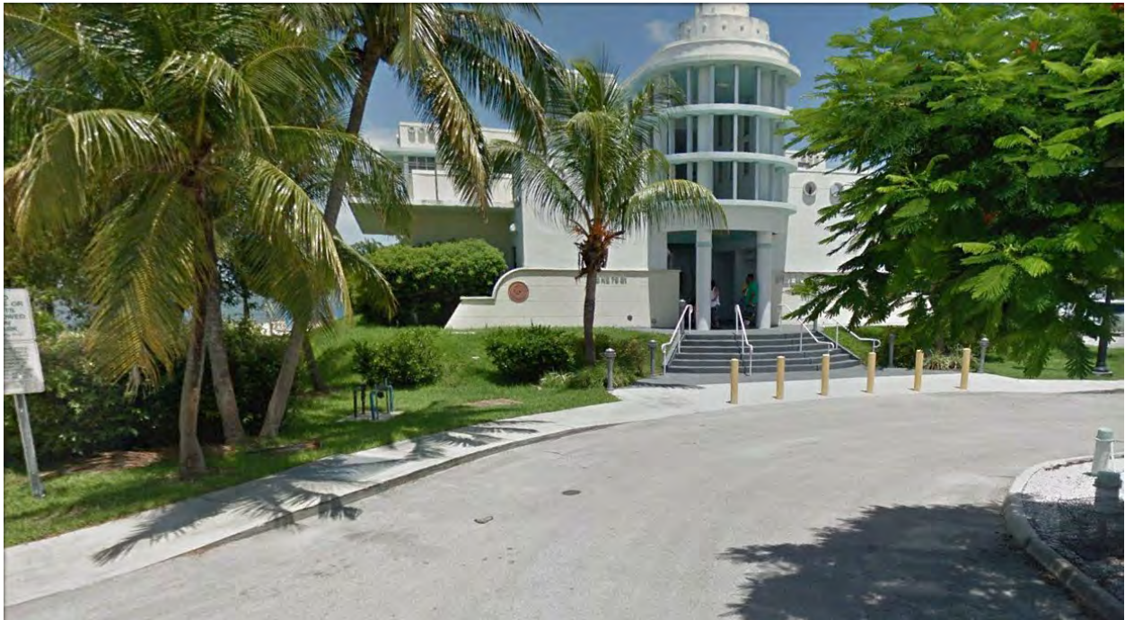
Photo 16 Marina Main Building, facing northeast
