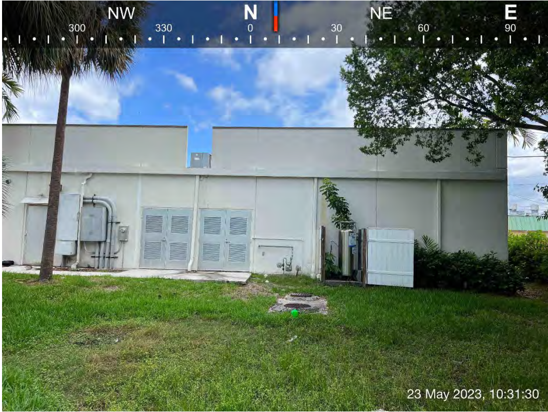
Photo 9 Back of gas station
