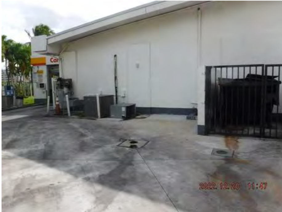
photo 3/4 - southeast view MW-9 & MW-9R
