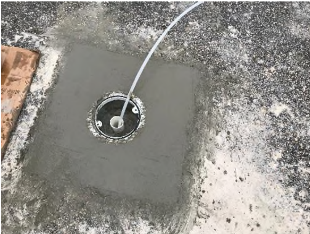
Photo 2 – View of monitoring well MW-M.
