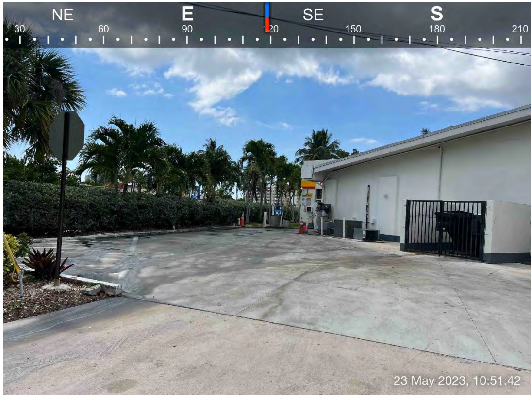
Photo 4 Back of gas station
