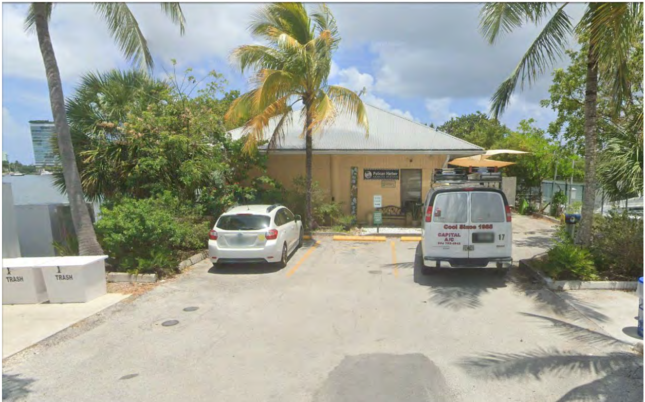
Photo 18 Ancillary Building at Marina, Facing South
