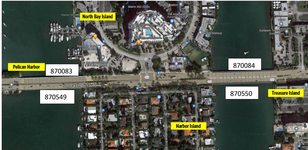
Figure 2.1 | Existing Bridge Structures
