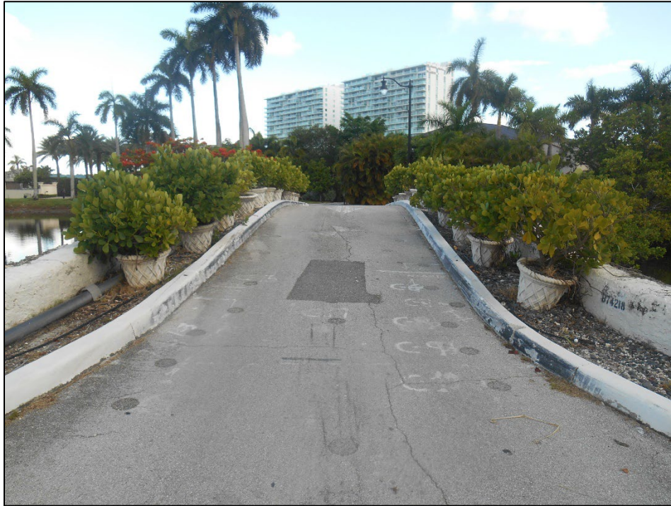
Figure 10-13 The Atlantic Island Bridge (8DA6433), c. 1925, determined National Register-eligible, facing North
