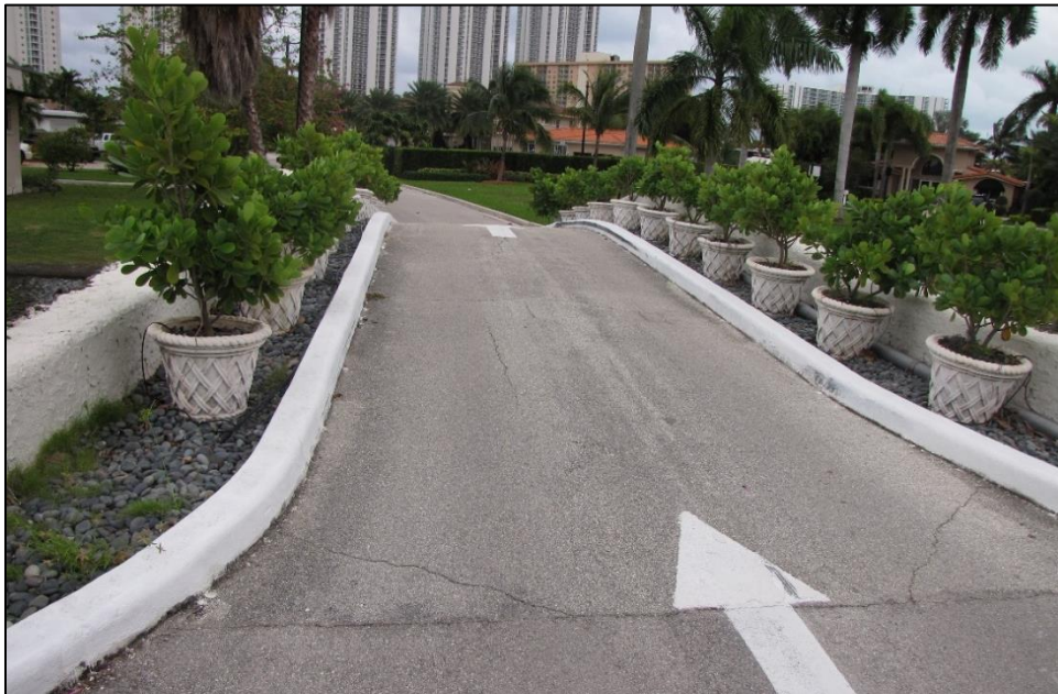
Figure 3: Deck of Atlantic Island Bridge/FDOT Bridge No. 874218 (8DA6433), Facing Southeast
