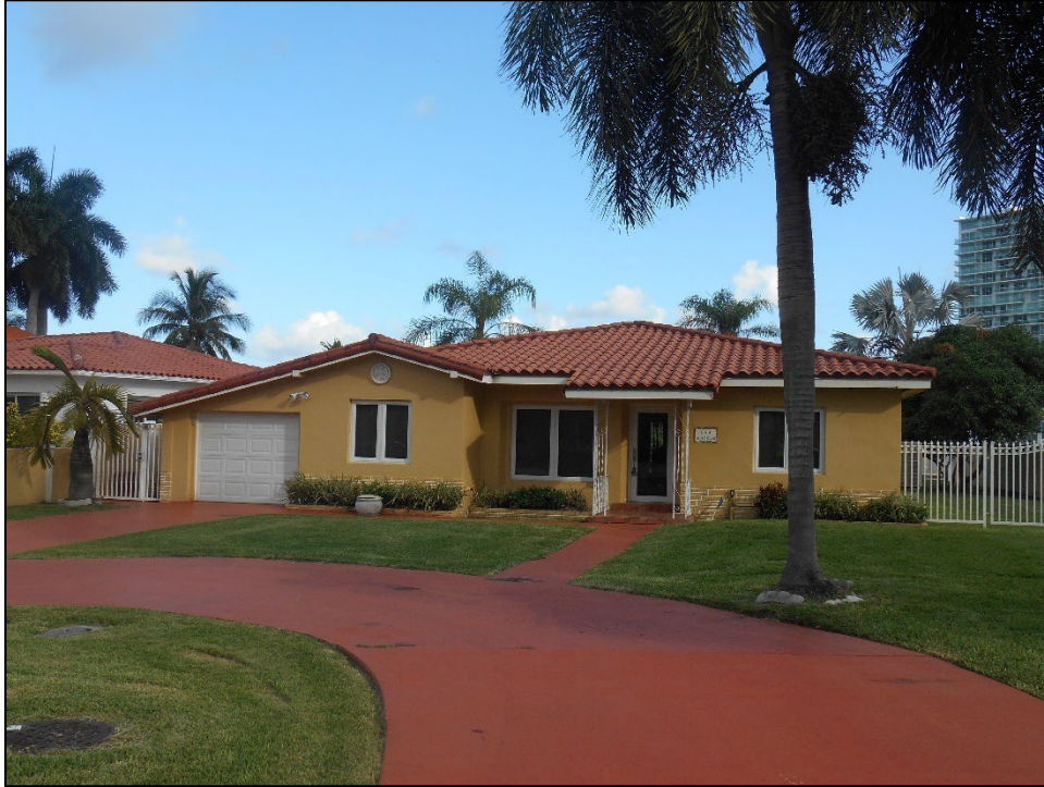
Figure 10-25 299 Atlantic Avenue (8DA19162), c. 1950, considered National Register-eligible, facing Northwest
