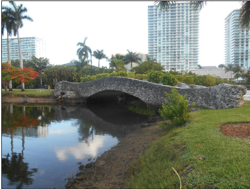
Figure 10-4 The Atlantic Island Bridge (8DA6433), c. 1925, determined National Register-eligible, facing Northeast
