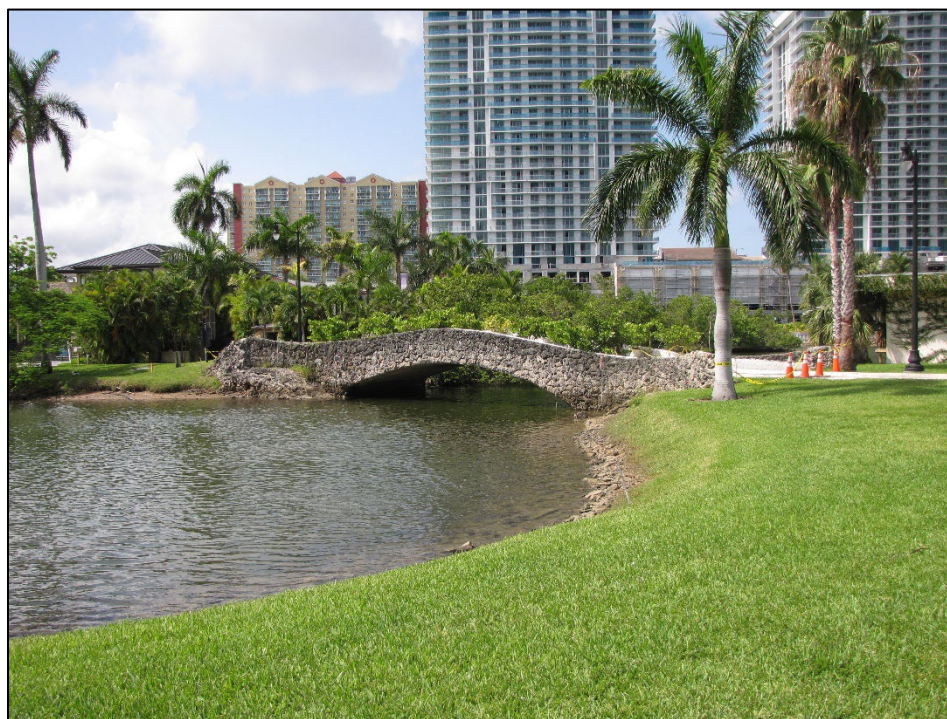
Figure 10-12 The Atlantic Island Bridge (8DA6433), c. 1925, determined National Register-eligible, facing East
