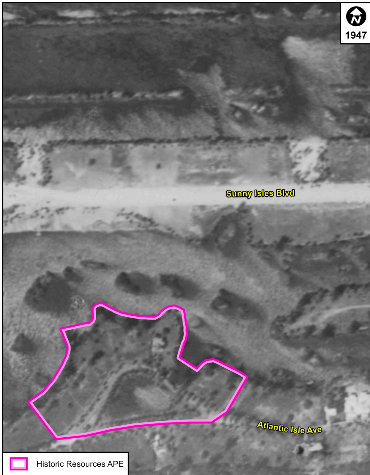
Figure 6-1 A 1947 historic aerial photograph of the Historic Resources APE
