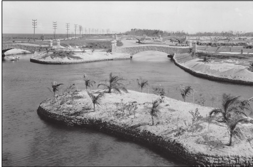
Figure 10-10 Historic photograph of the entrance bridges to the Atlantic Island development ( Obtained from Bramson )
