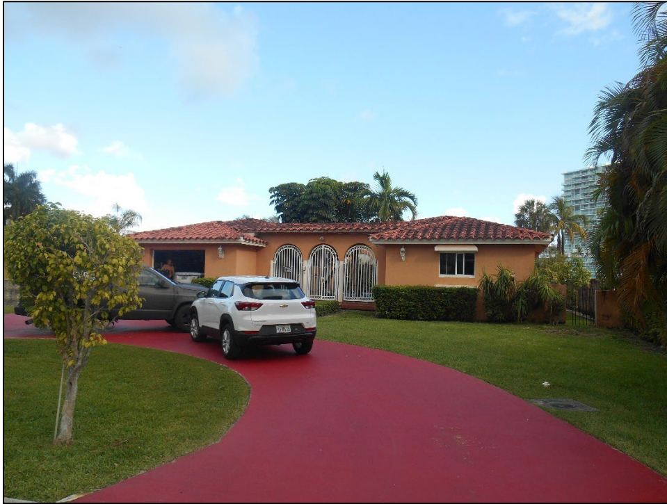
Figure 10-24 291 Atlantic Avenue (8DA19161), c. 1970, considered National Register-ineligible, facing Northwest
