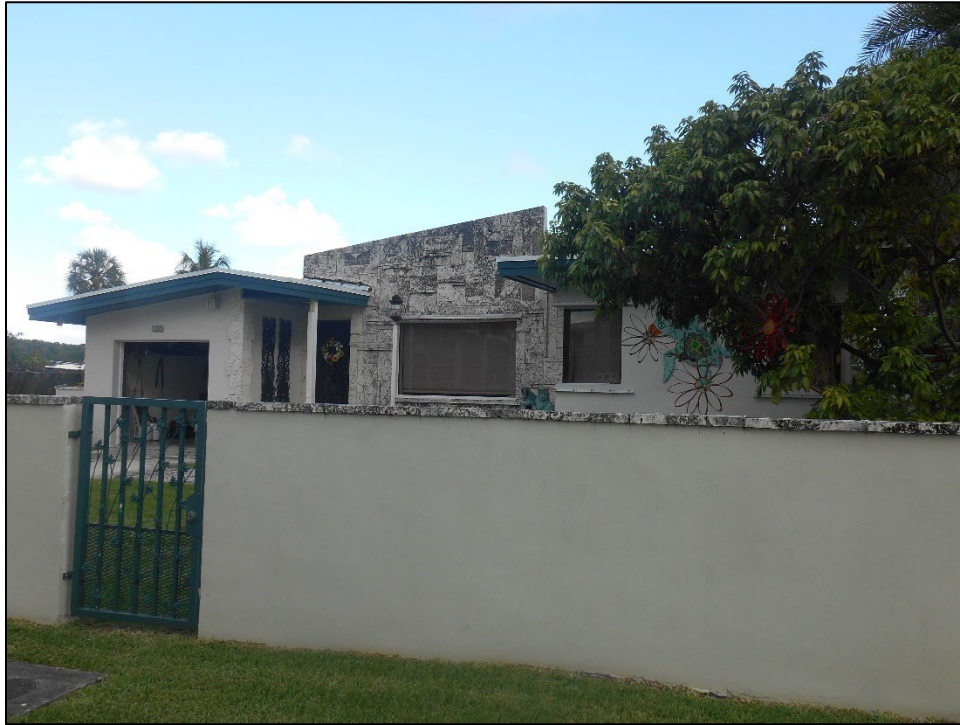
Figure 10-23 283 Atlantic Avenue (8DA19160), c. 1951, considered National Register-eligible, facing Northwest
