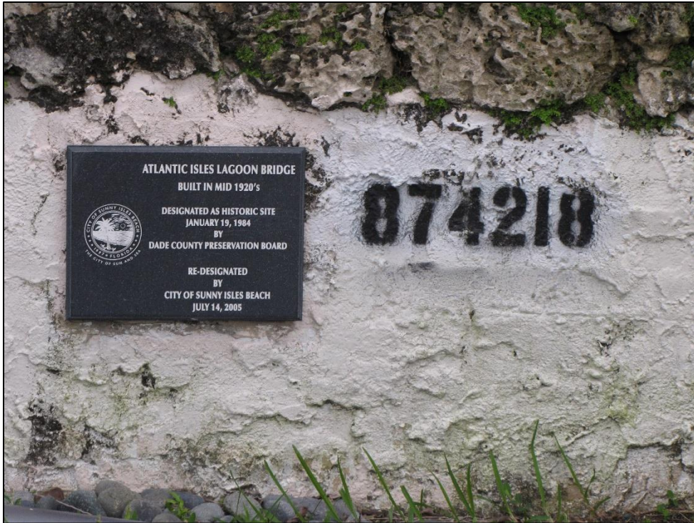
Figure 5: Plaque Designating Atlantic Island Bridge/FDOT Bridge No. 874218 (8DA6433) as a Local Historic Landmark, Facing South
