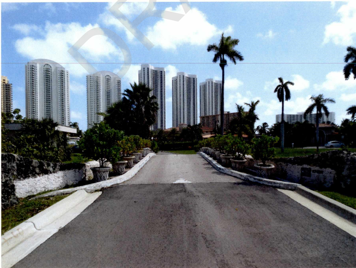
EAST APPROACH OF BRIDGE
