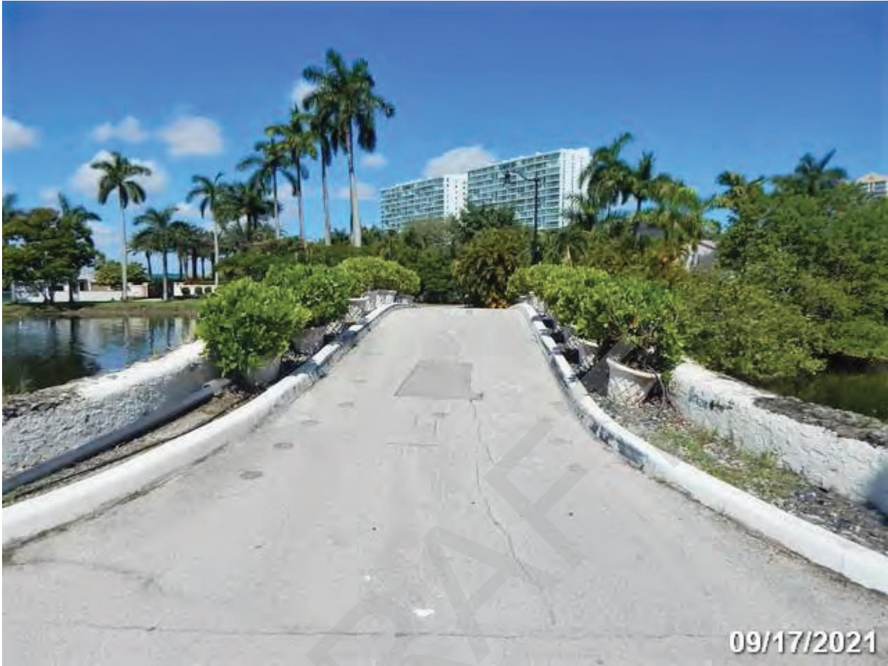
East Approach Looking West - 09/17/2021
