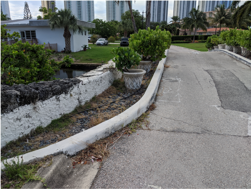
Figure 9: Planter Area – Typical on both Sides of Bridge
