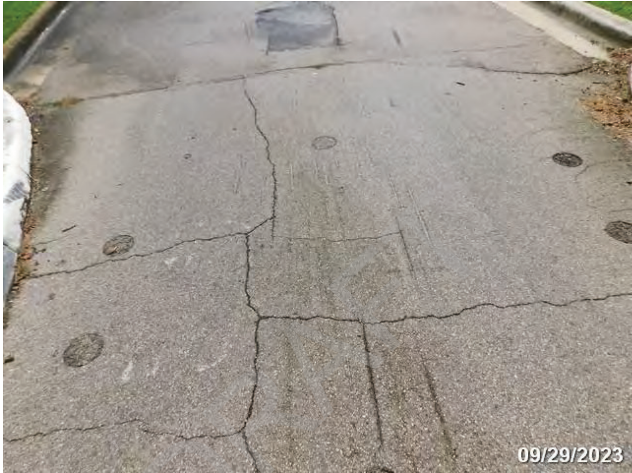
PHOTO 6: ELEMENT/ENV: 144/4 Re Conc Arch
