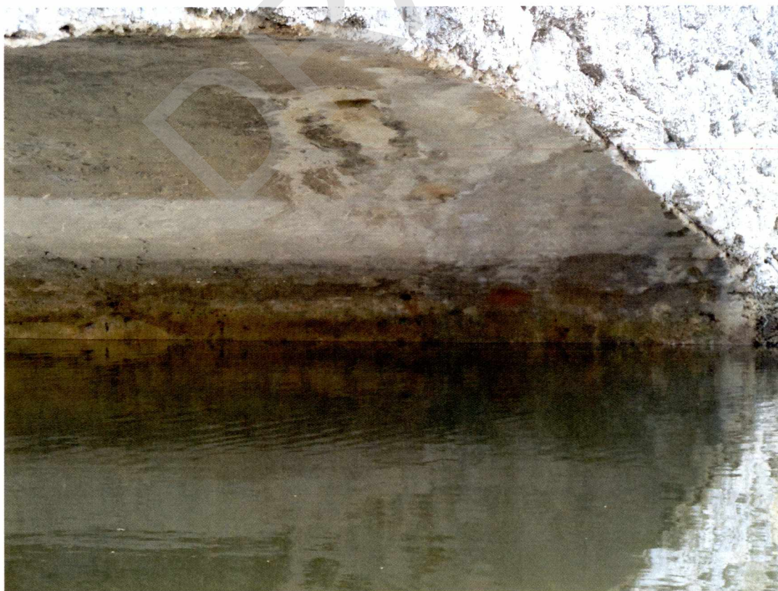
UNDER BRIDGE VIEW
