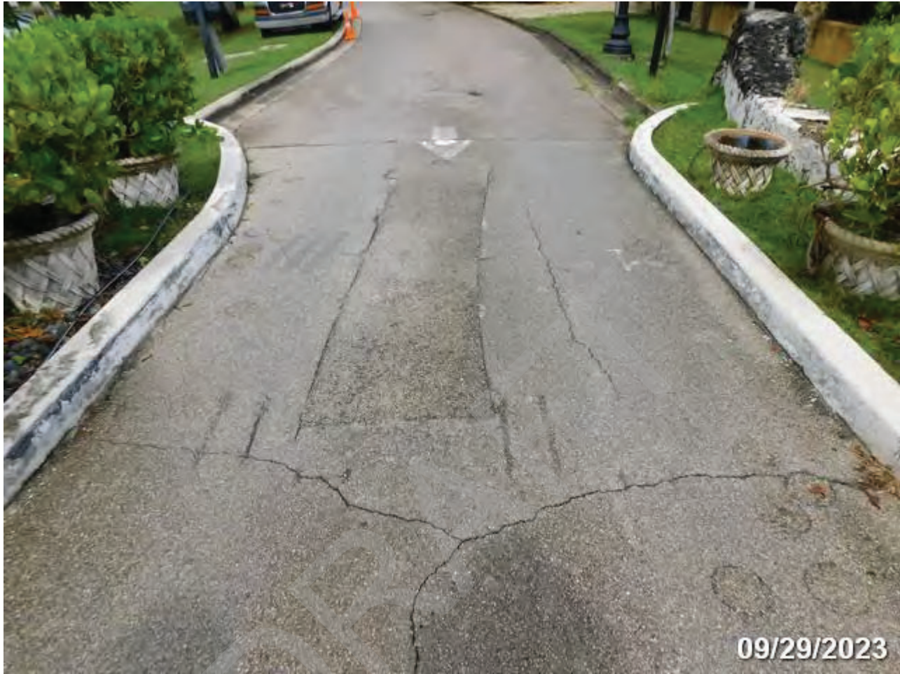
PHOTO 5: ELEMENT/ENV: 144/4 Re Conc Arch
