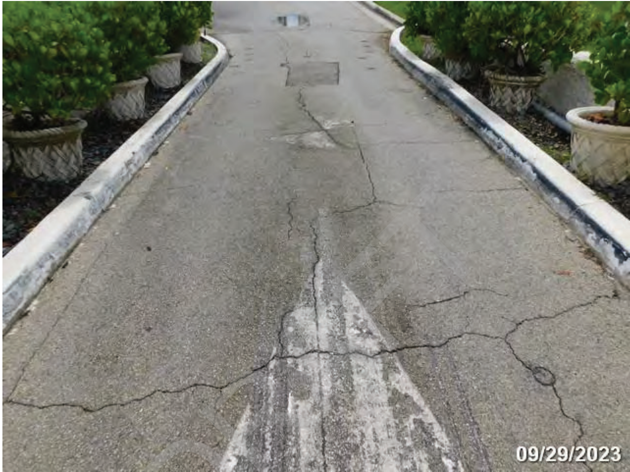
PHOTO 4: ELEMENT/ENV: 144/4 Re Conc Arch
