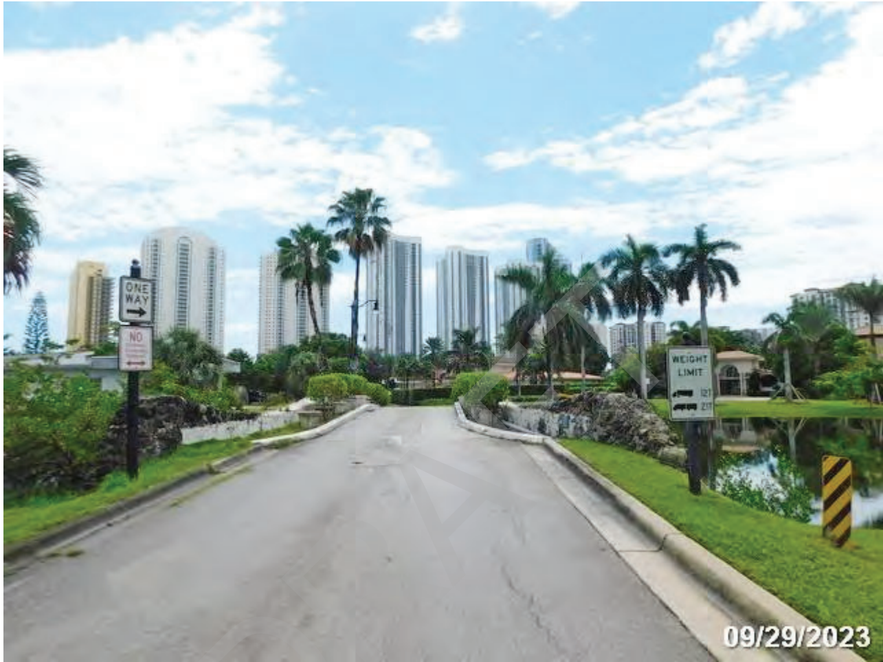
PHOTO 8: ELEMENT/ENV: 144/4 Re Conc Arch
