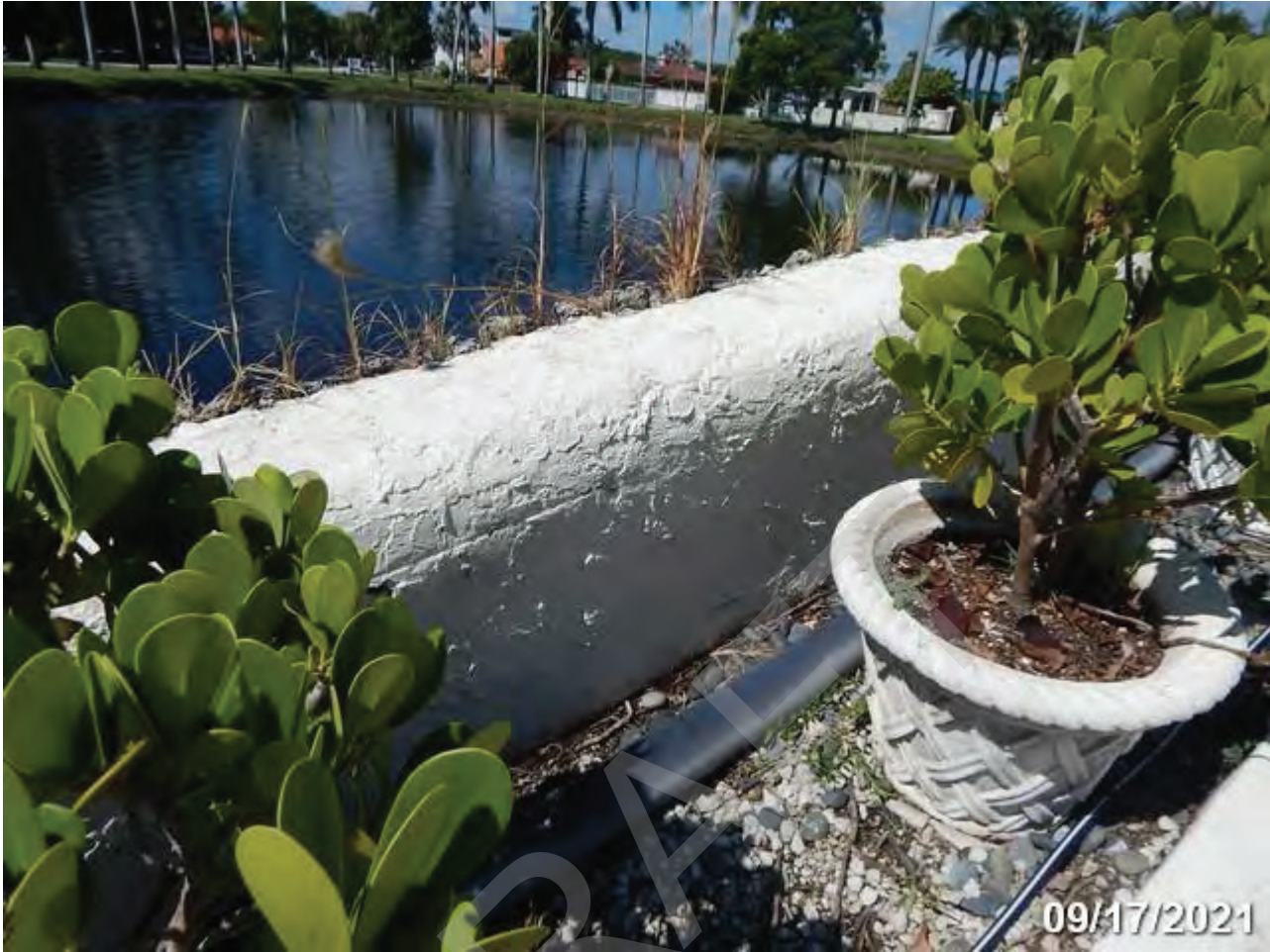
Typical Bridge Rail - 09/17/2021
