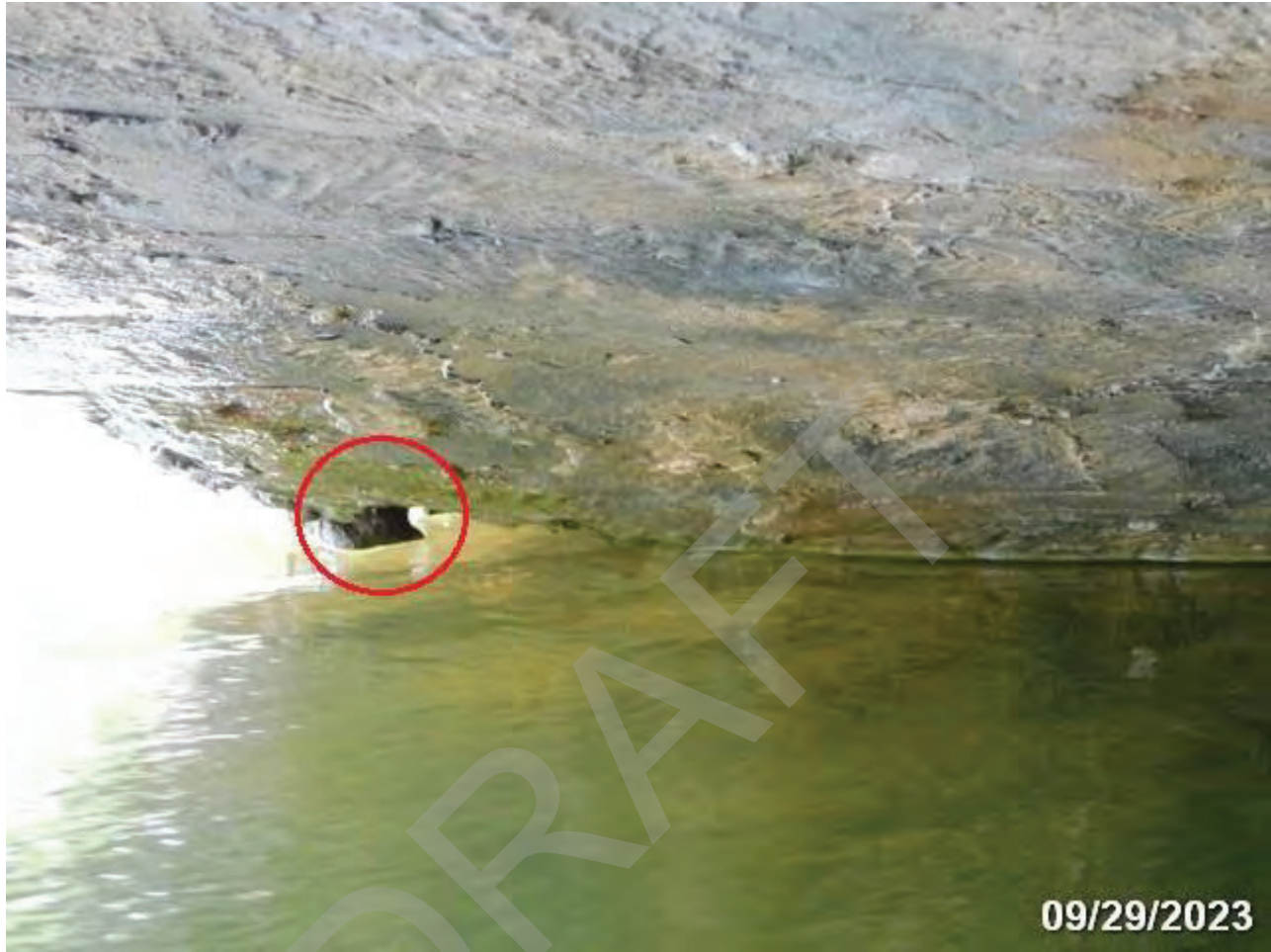
PHOTO 12: ELEMENT/ENV: 144/4 Re Conc Arch
