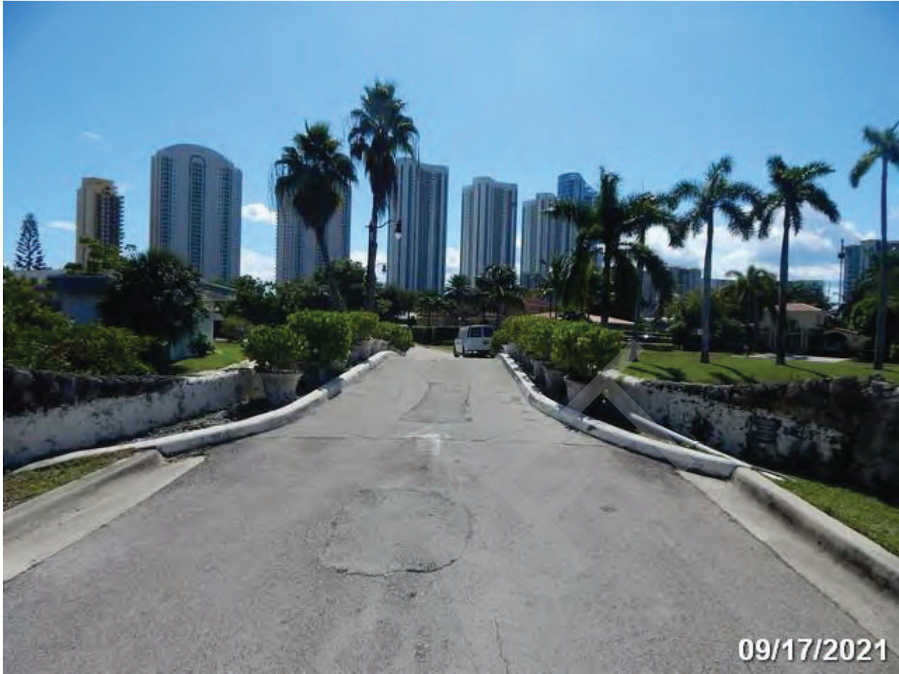
West Approach Looking East - 09/17/2021
