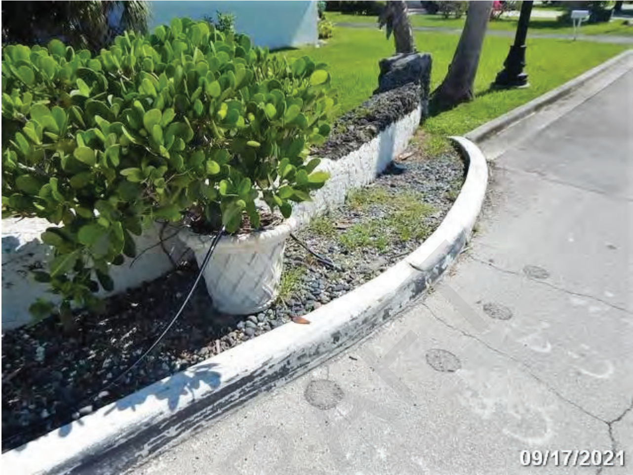
Northeast Off-Going Transition - 09/17/2021
