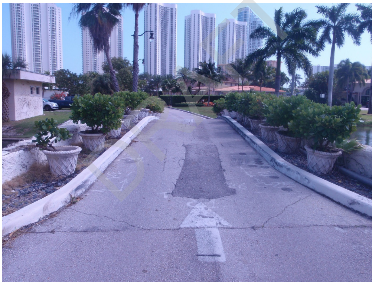
Figure 2-9. Existing Planter Easement Along Bridge
