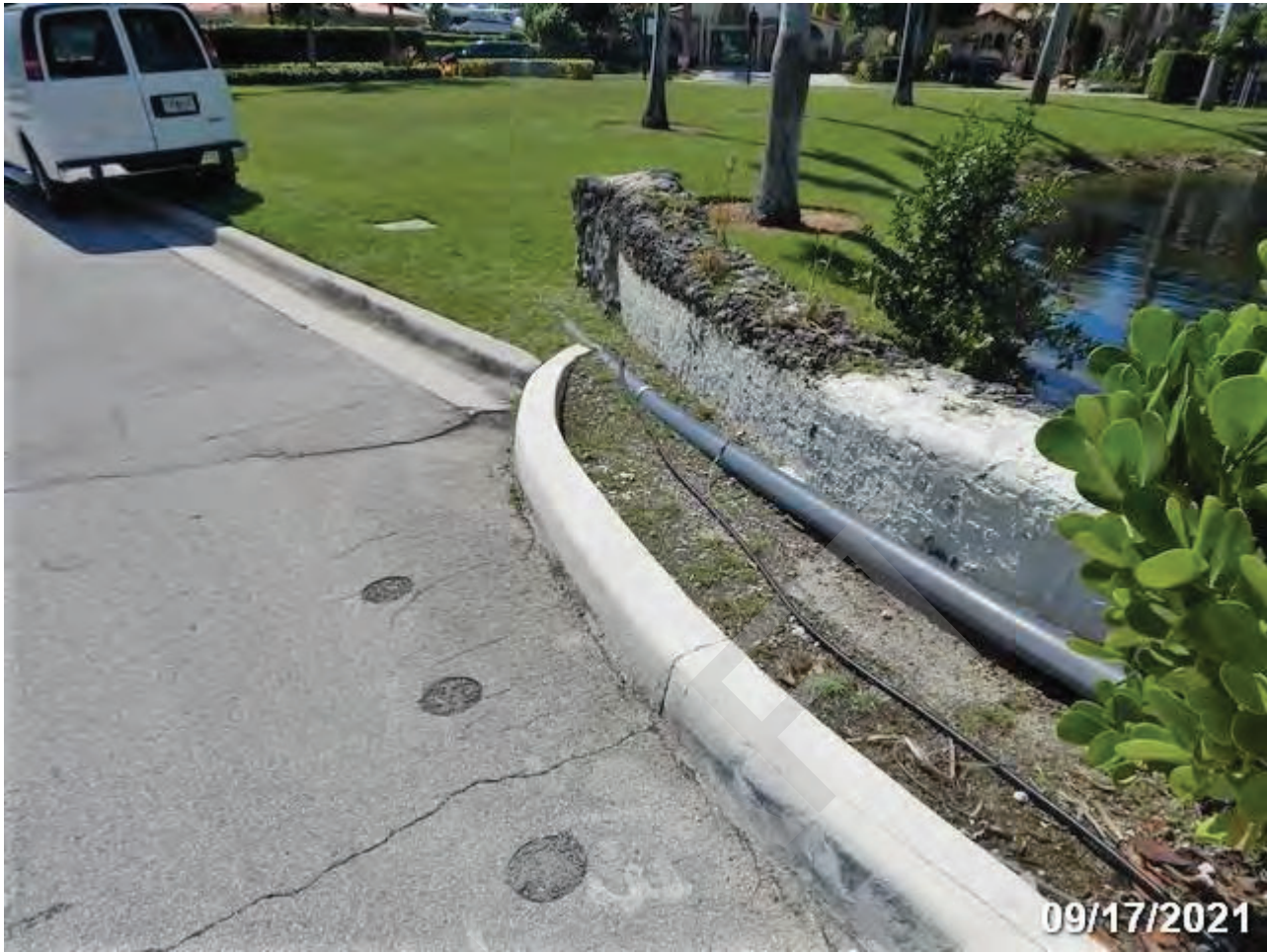
Southeast Off-Going Transition - 09/17/2021
