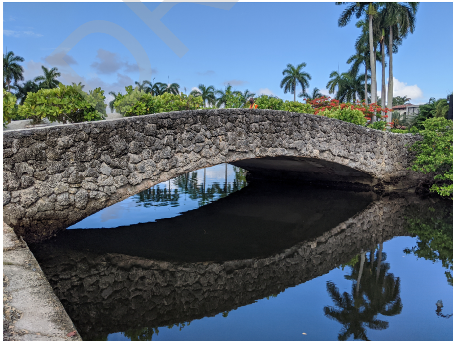
Figure 4: Overall Bridge Elevation View – Looking Southwest
