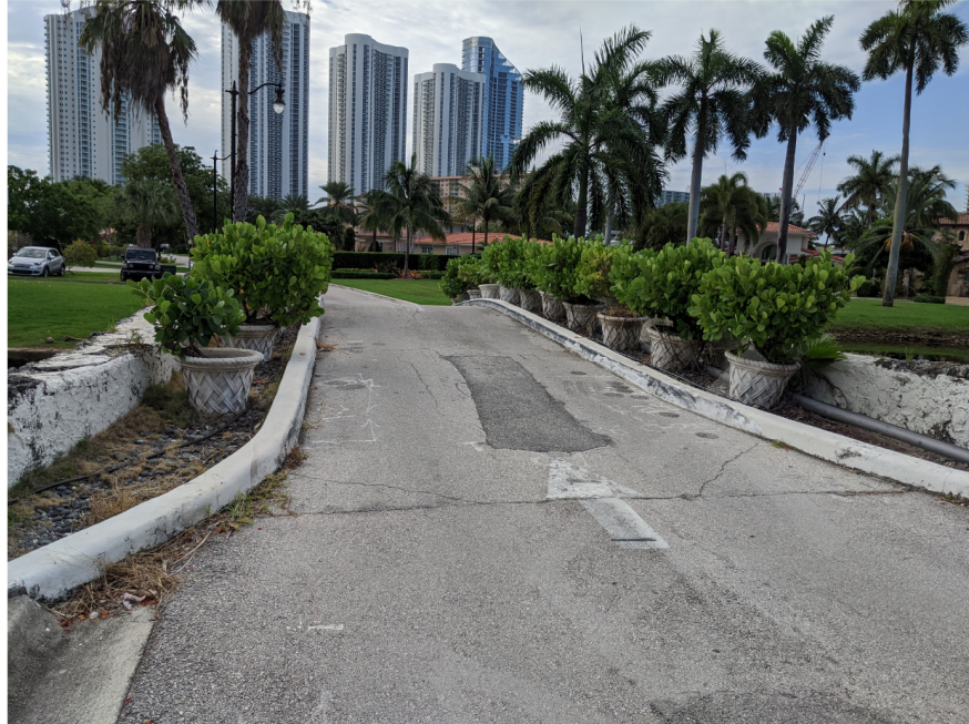
Figure 3: Overall Bridge Deck View – Looking East
