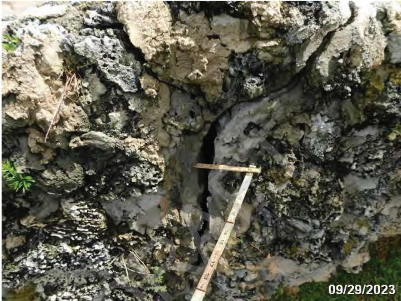
PHOTO 2: ELEMENT/ENV: 8477/4 Other Wingwalls/Retaining Wall
