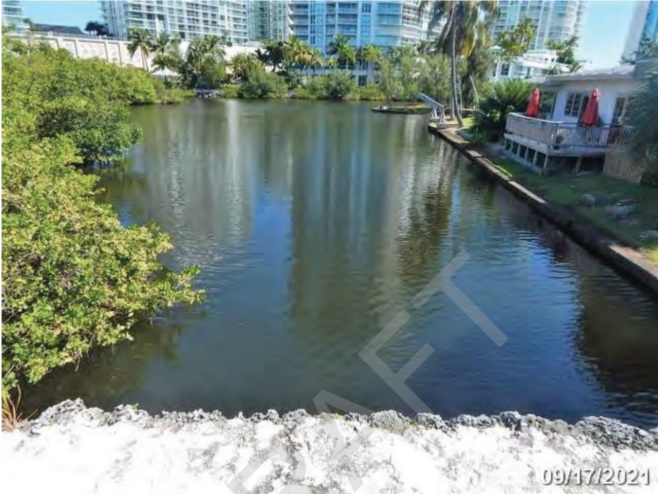
Channel Looking North - 09/17/2021
