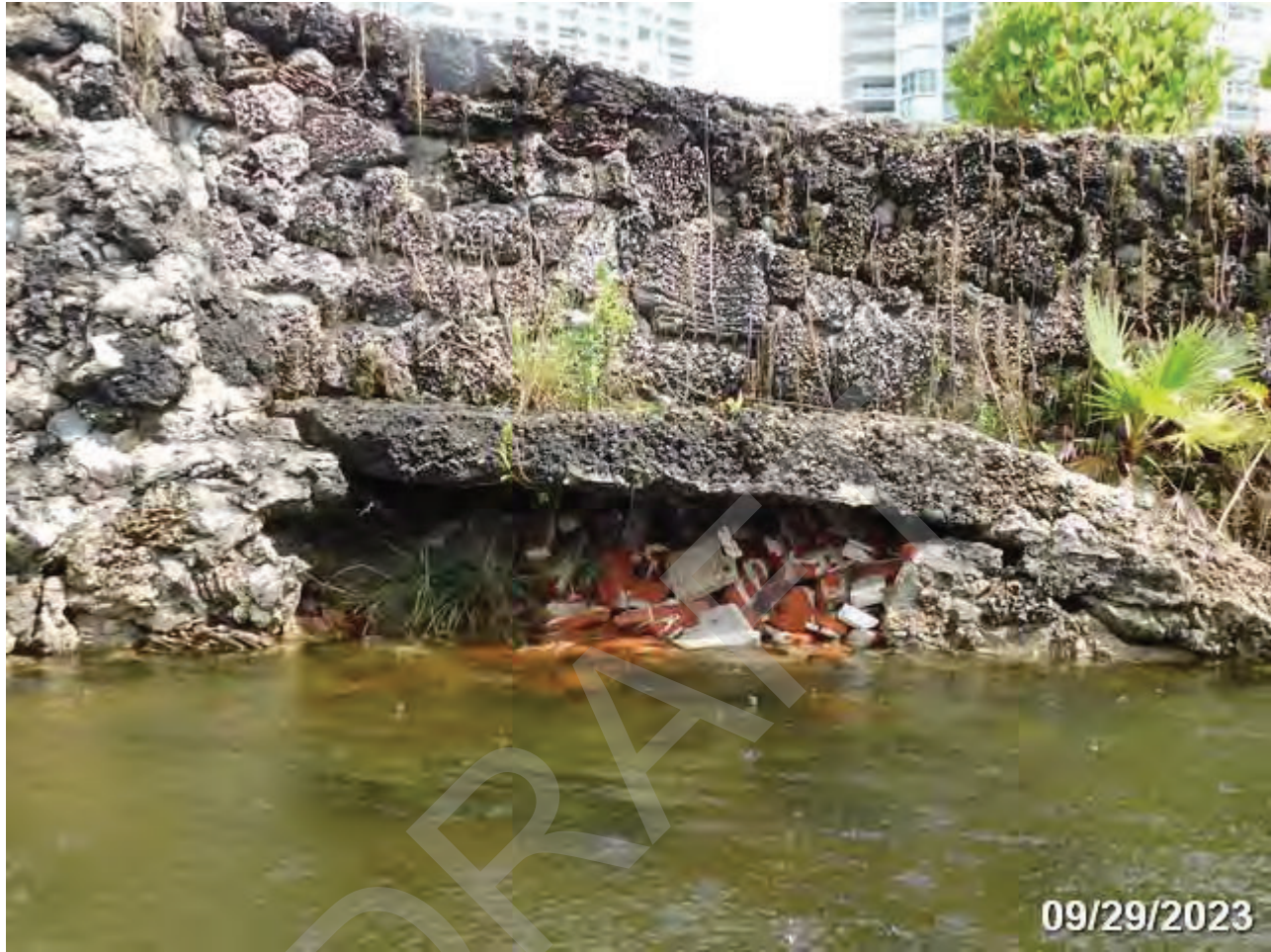
PHOTO 3: ELEMENT/ENV: 8477/4 Other Wingwalls/Retaining Wall
