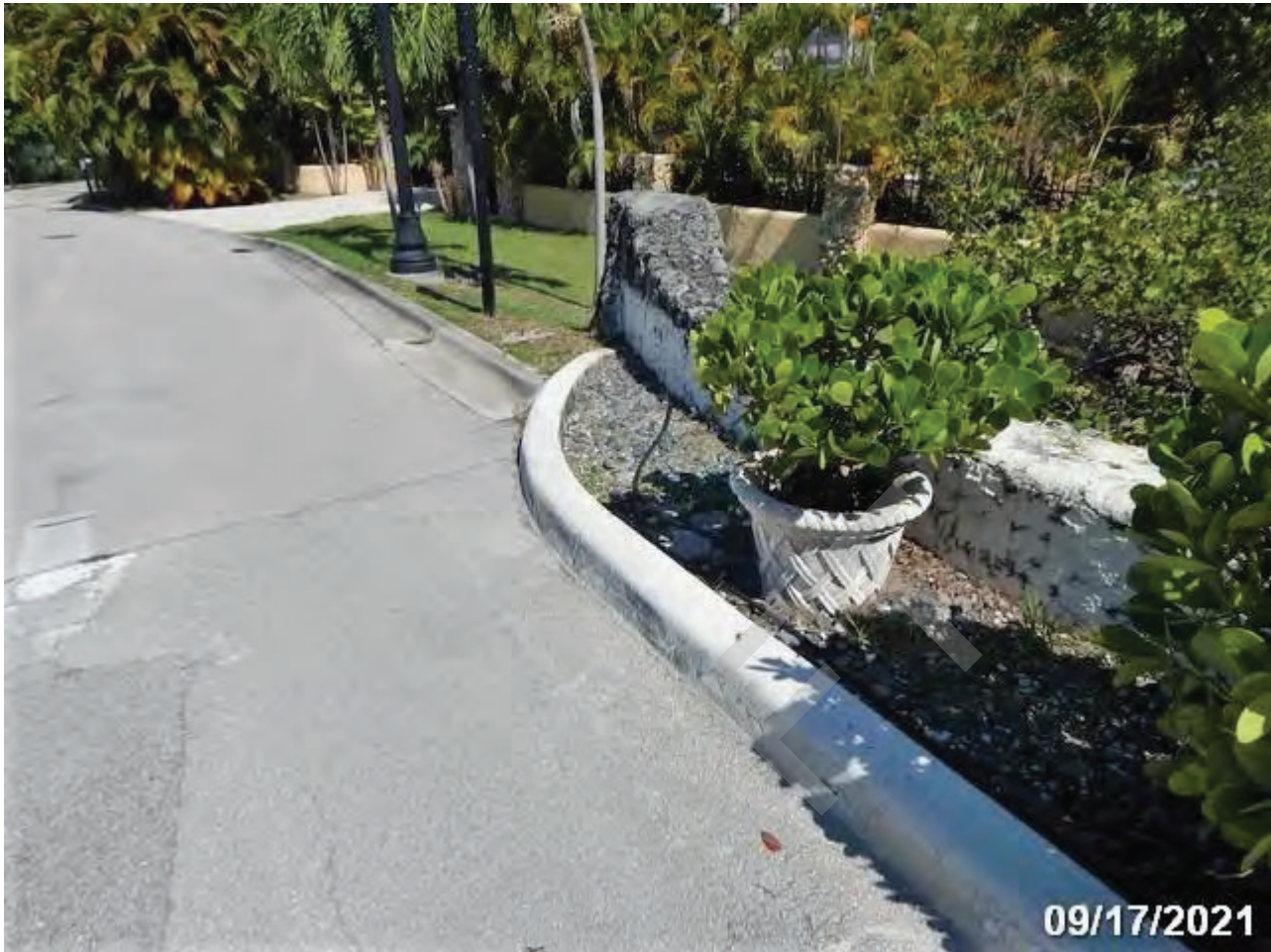
Northwest Oncoming Transition - 09/17/2021
