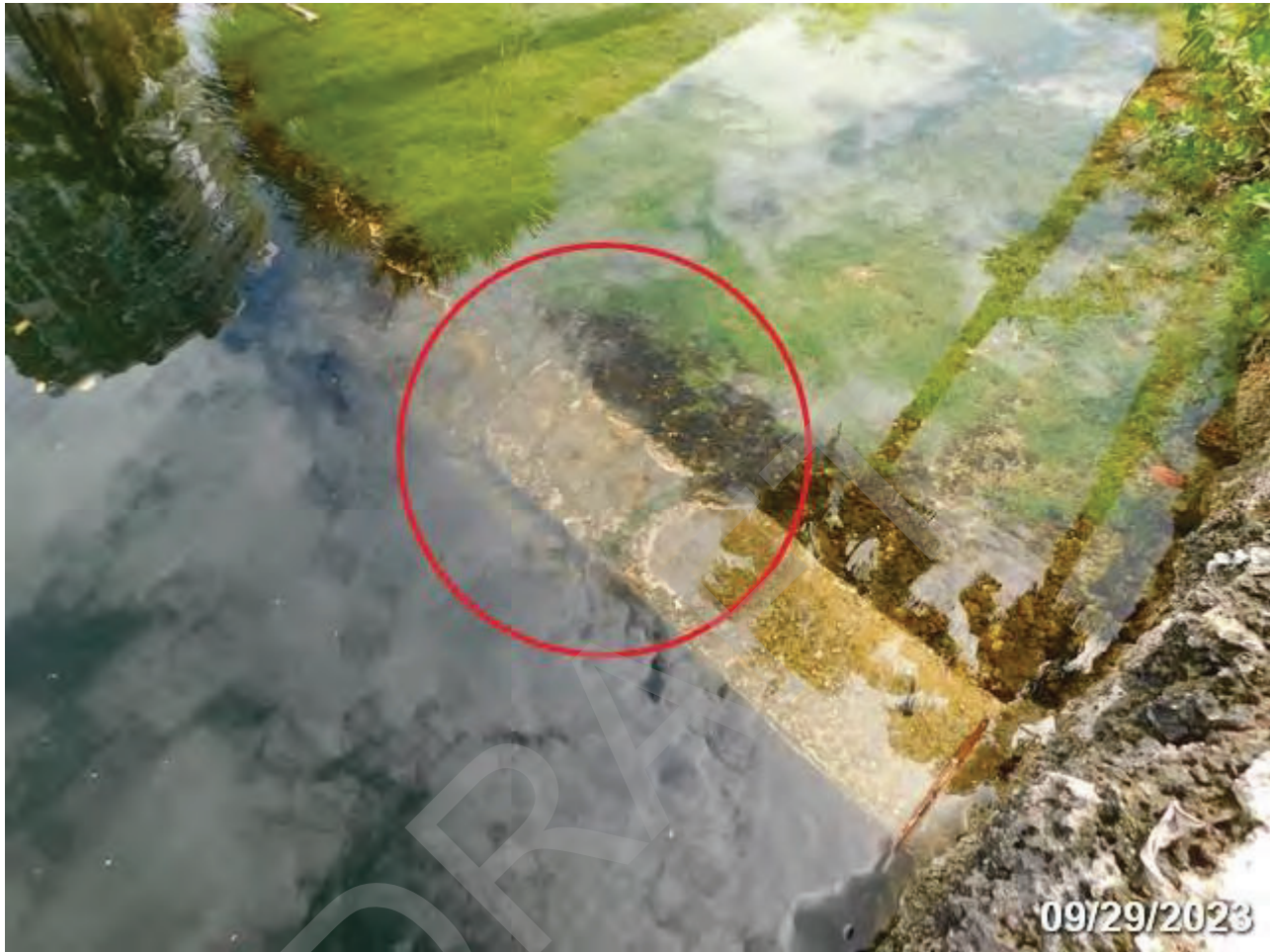
PHOTO 1: ELEMENT/ENV: 8477/4 Other Wingwalls/Retaining Wall
