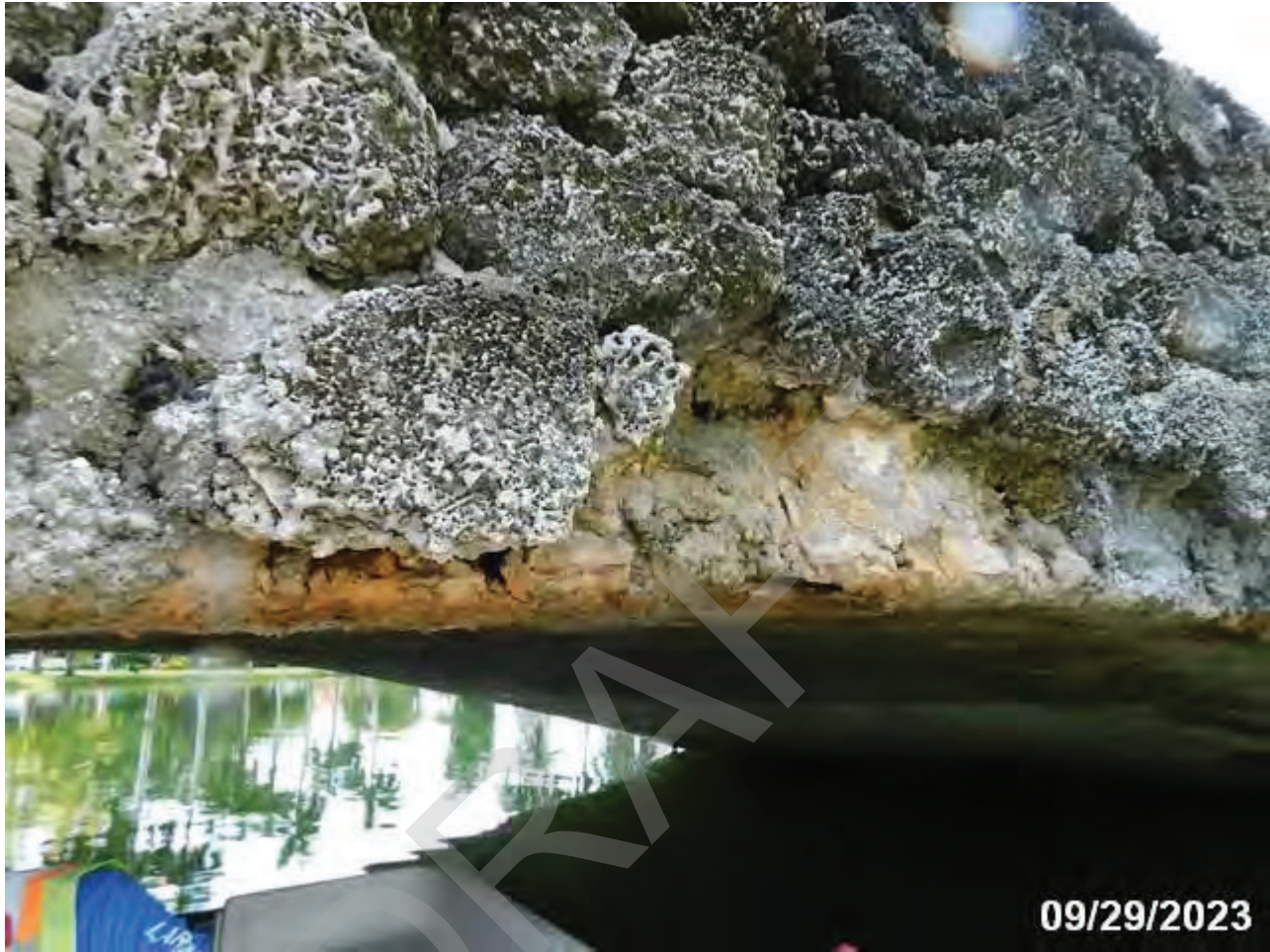
PHOTO 7: ELEMENT/ENV: 144/4 Re Conc Arch
