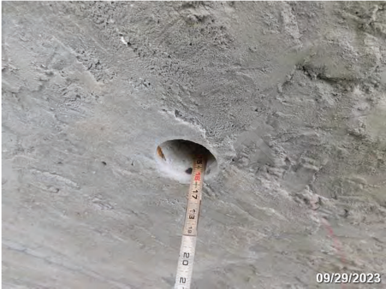
PHOTO 11: ELEMENT/ENV: 144/4 Re Conc Arch
