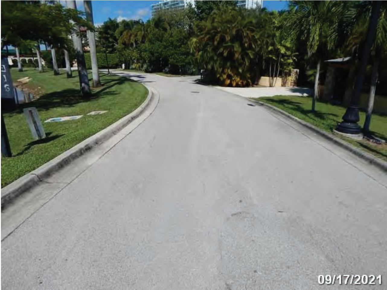
West Approach Looking West - 09/17/2021
