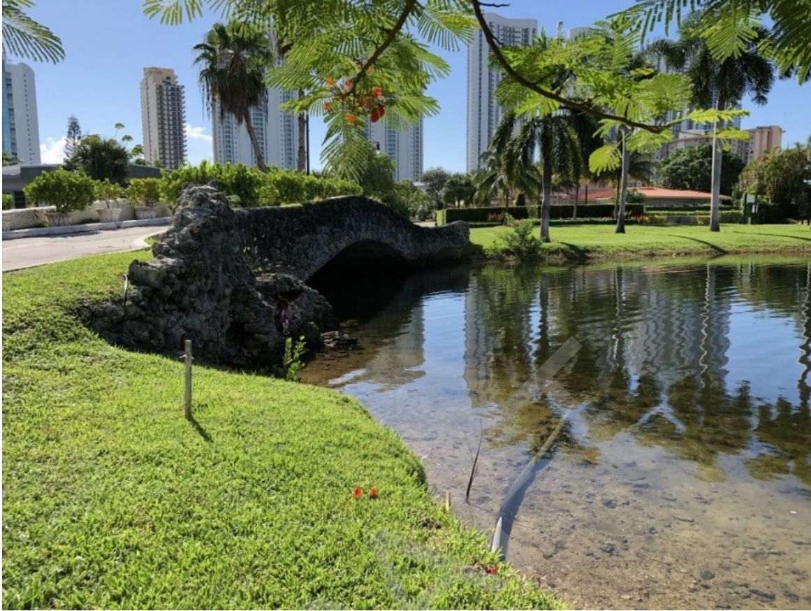
Figure 2-12. Atlantic Isle Lagoon Bridge – Southeastern View
