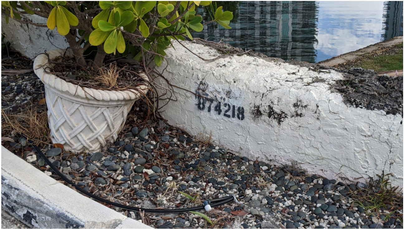
Figure 7: Bridge Number on Northern Parapet
