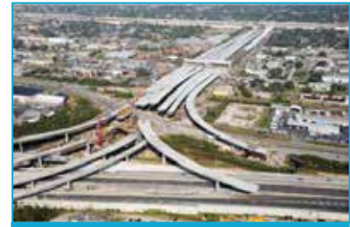
COMPLEX SEGMENTAL URBAN VIADUCTS (I-4 CONNECTOR)
