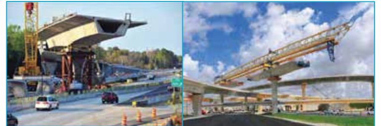
Ground-Base Crane Overhead Gantry BALANCED CANTILEVER CONSTRUCTION
