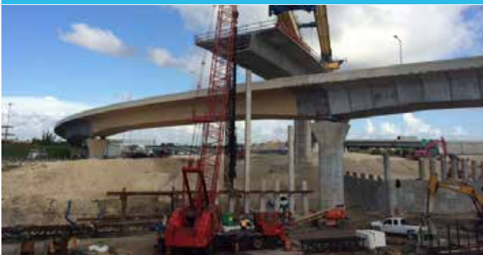
PILE DRIVING OPERATIONS
