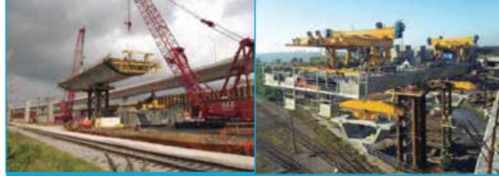
CRANE & SPECIALIZED SEGMENT LIFTERS TO ERECT OVER CSX RR
