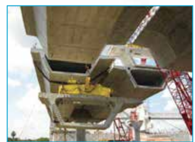
ERECTION ON ADJACENT BOX GIRDERS WITH TRANSVERSE POST-TENSIONING
