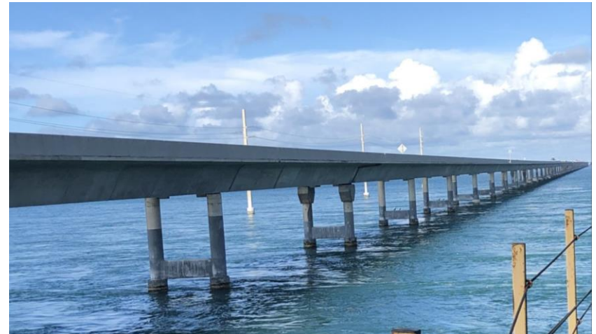
Seven Mile Bridge
