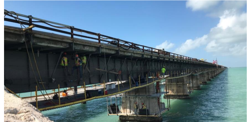
Old Seven Mile Bridge Steel Operations and Concrete Spall Repairs
