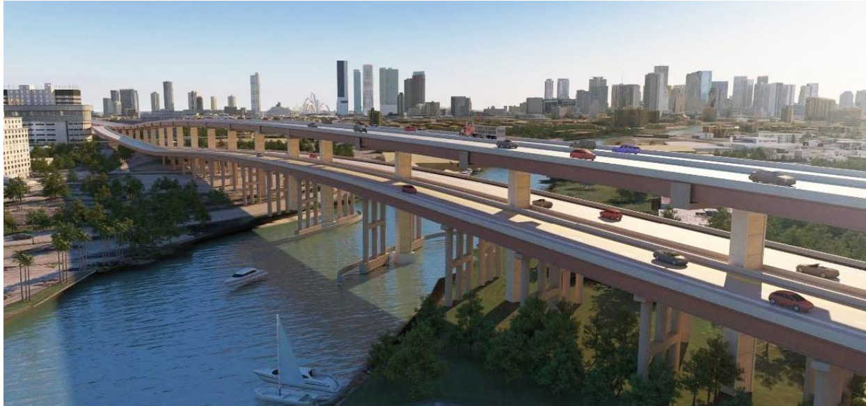
SR 836 Viaduct over the Miami River
